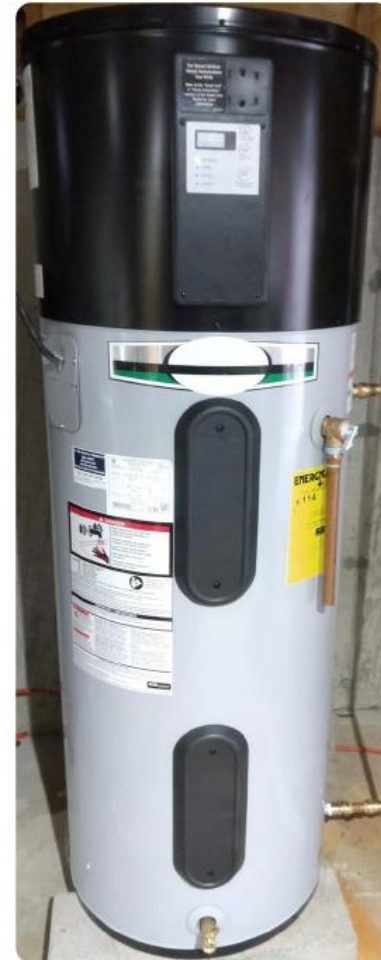
Heat Pump Water Heater
